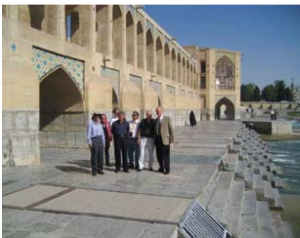
Figure 1. Magnificent Isfahan, the famous Khaju Bridge over the Zayandeh River, built in 1650 by Shah Abbas II, with intersecting arches and sluice gates that regulate water flow.
