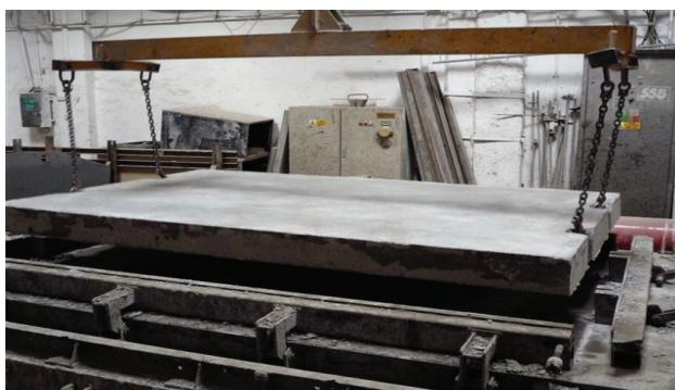
Figure 21 Remoulding a precast concrete with waste polyurethane foam unit after 24 hours
