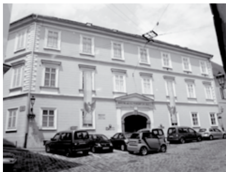
Figure 11. Museum building in Demetrova which the institution has occupied since 1866 until today.
