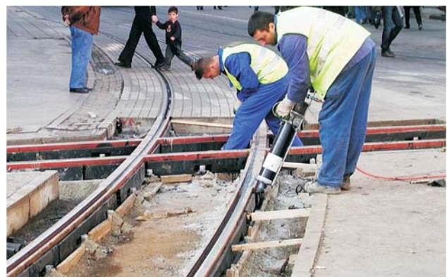
Figure 5 Infusion of elastomeric material between discrete supports
