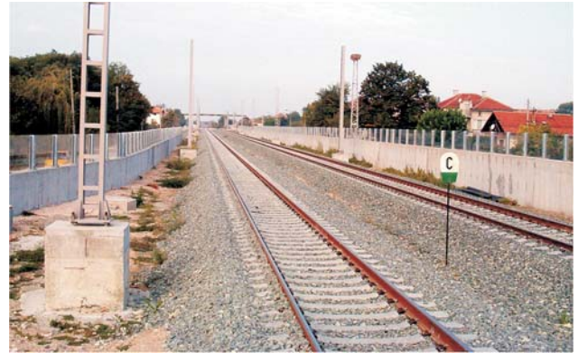
Figure 25 Noise protection barrier
