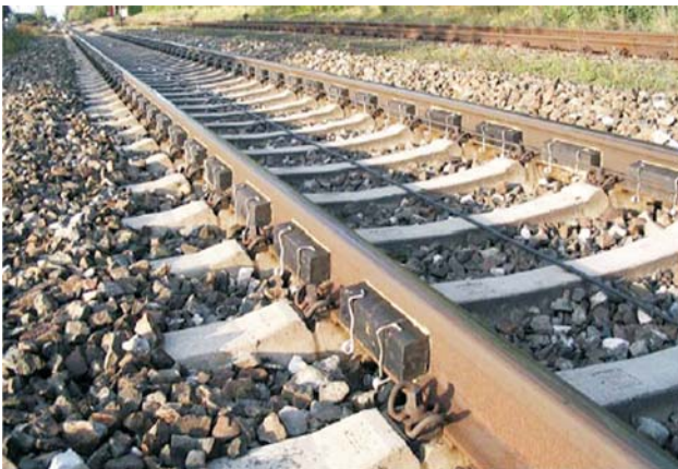
Figure 8 Rail vibration dampers
