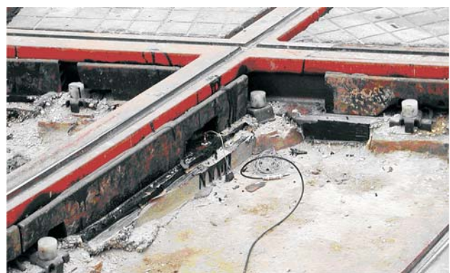
Figure 6 Continuously supported and embedded rail
