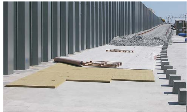
Figure 13 Sub-ballast mat
