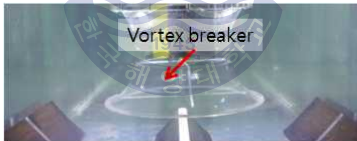
(b) Vortex breaker installation
