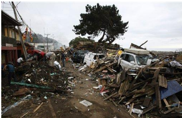
(a) Damage by the tsunami
