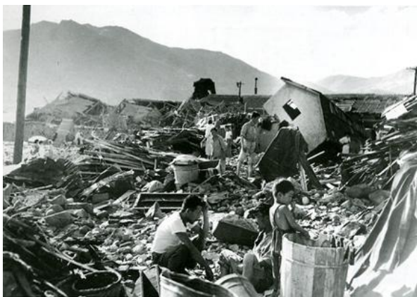
(a) Damages by typhoon Sarah
