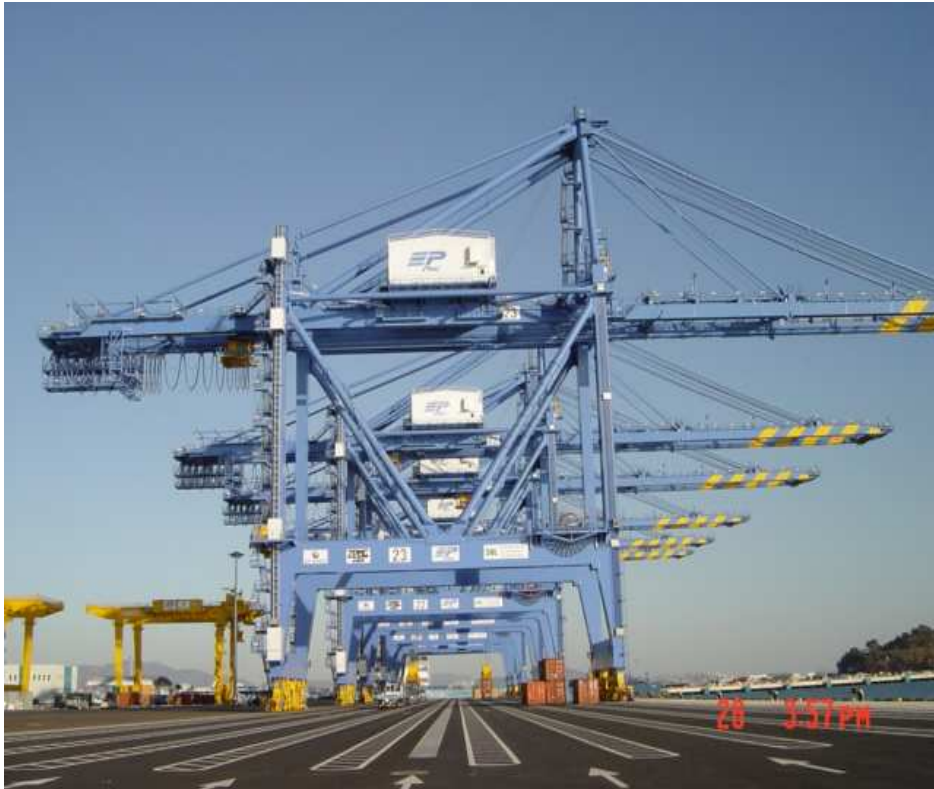
Fig. 2.3 A view of gantry crane
