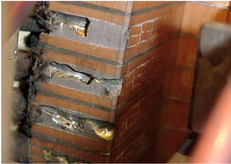
Fig. 3.6 Faults of DC motor
