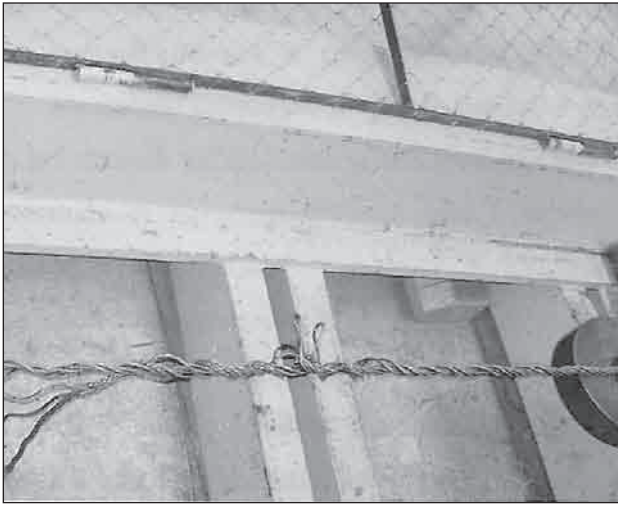
Figure 7 Ruptured steel wire rope. Same rope (figure 6) in visible light.
