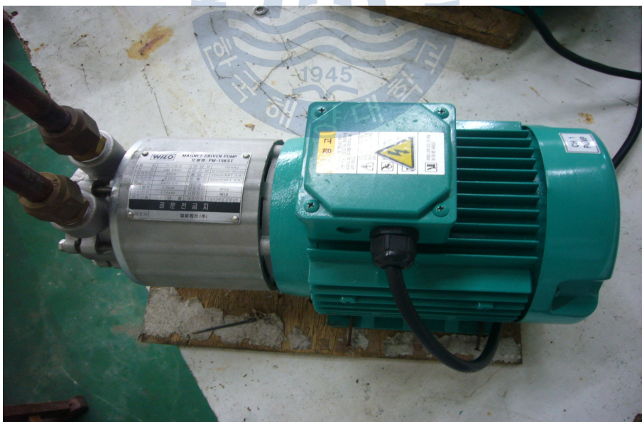
Fig. 3.20 Refrigerant pump
