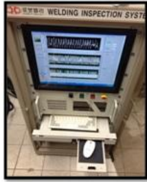
Welding inspection system
