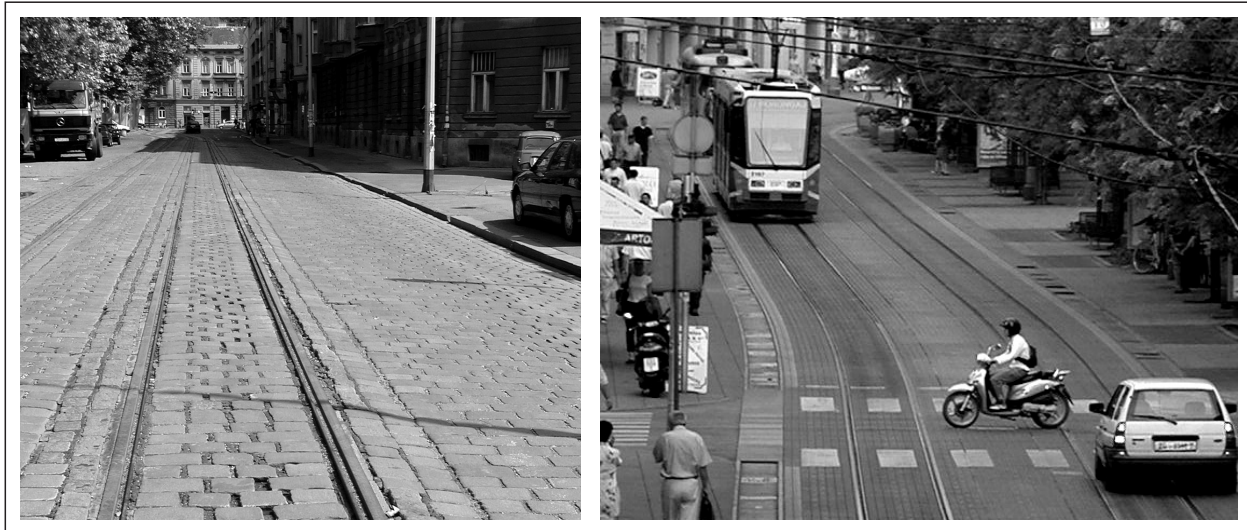
Figure 5 - Survey of tram track embedded in road surface
