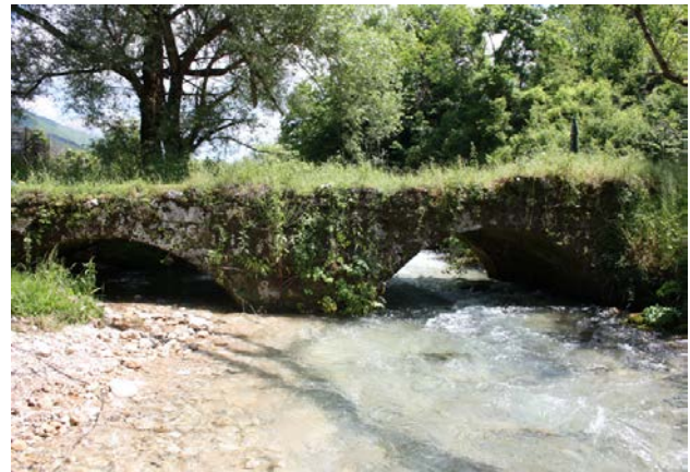
Figure 4 - San Teodoro Bridge gauging section (ST_01)
