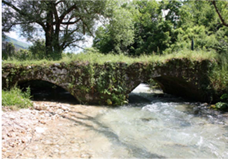
Figure 5.9 San Teodoro Bridge gauging section (SW_04)
