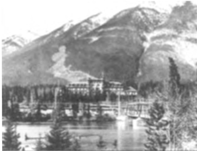
FIGURE 3. The Sanitarium (part hospital, part poolroom, and part bar) was built by Dr. Brett in 1887. Fire destroyed the building in 1892 and the Park Administration building now stands in its place.
