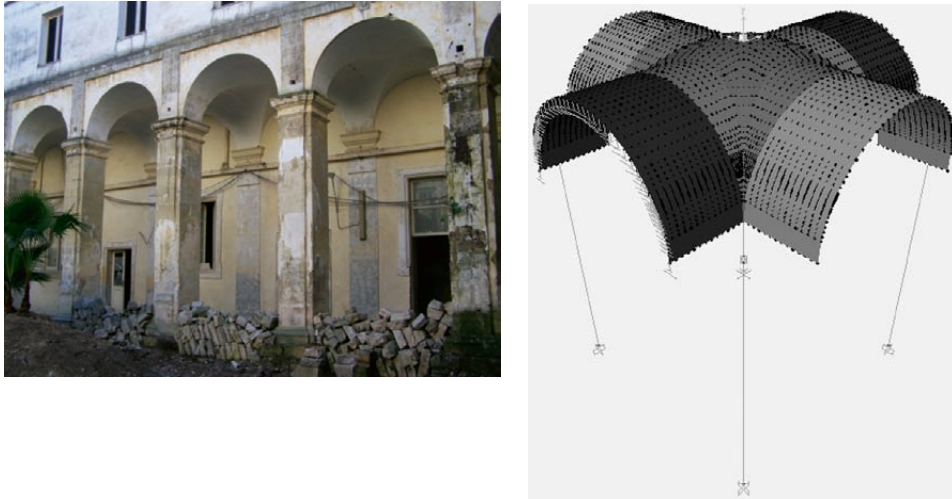
Figure 9. External view of the central cloister ( left ) and FE model of the masonry cell ( right ).
