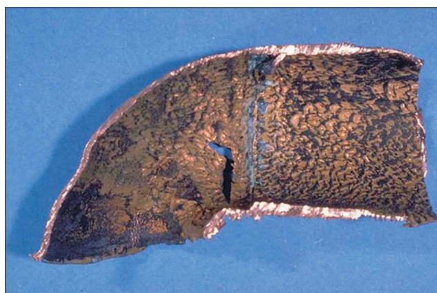
Fig. 4. The "Horseshoe" type erosion-corrosion damage in a copper pipeline.
