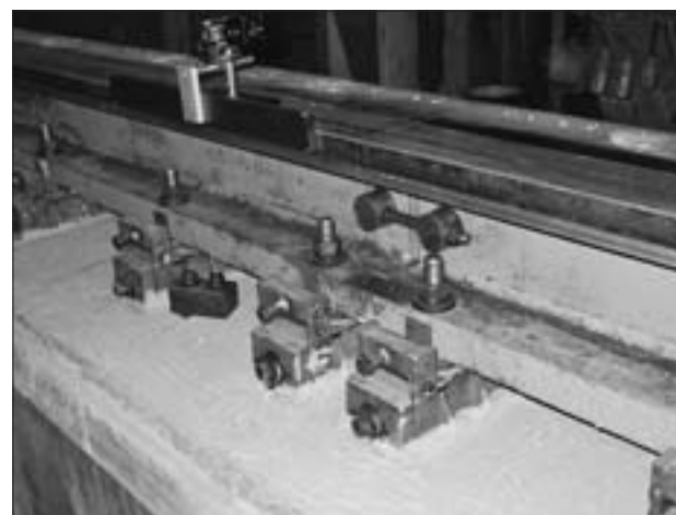
Figure 1 The way of fixing the guideway to the ground and joining two segments
