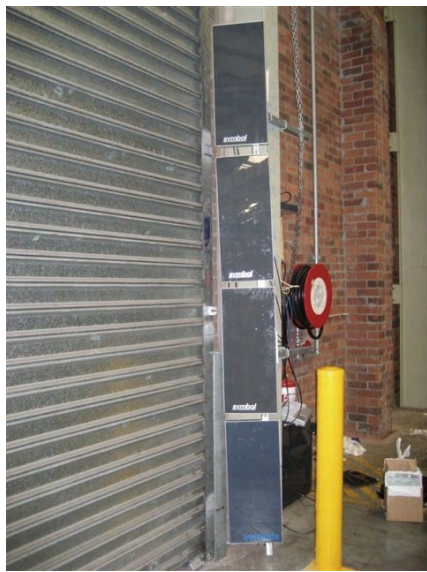
Fig. 6. Antennae mounted as one-sided configuration
