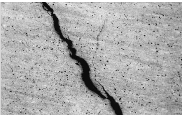
Figure 4 Parallel cracks (OM); magnification 100x.
