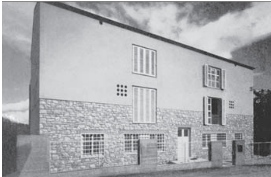
SL. 5. VILA MEIXNER, ZAGREB, MALLINOVA ULICA 14, ZAPADNO PROČELJE FIG. 5 VILLA MEIXNER, ZAGREB, 14 MALLINOVA STREET, WEST FAÇADE
