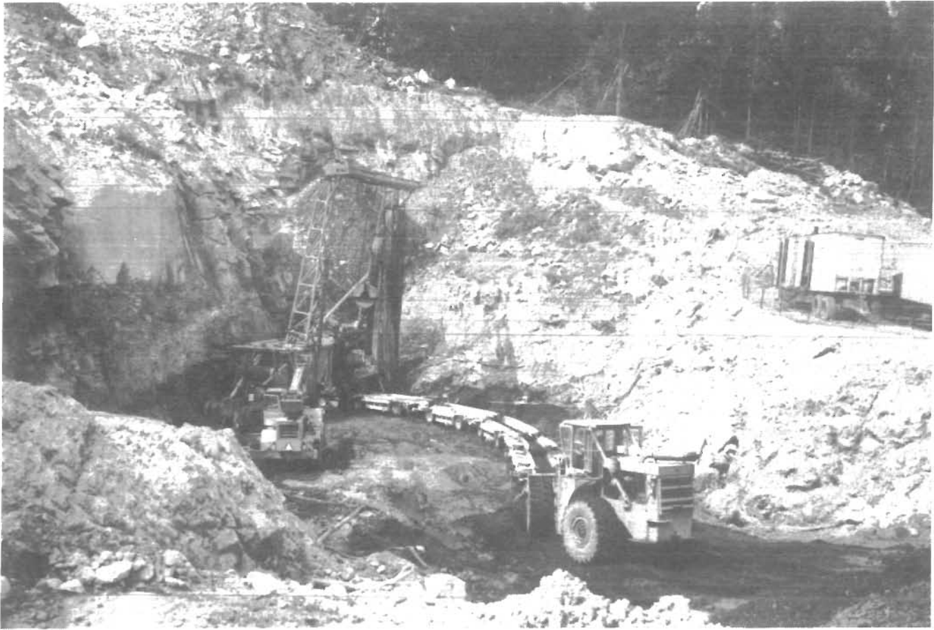
Figure 13.—Teleoperated highwall mining system at production site.
