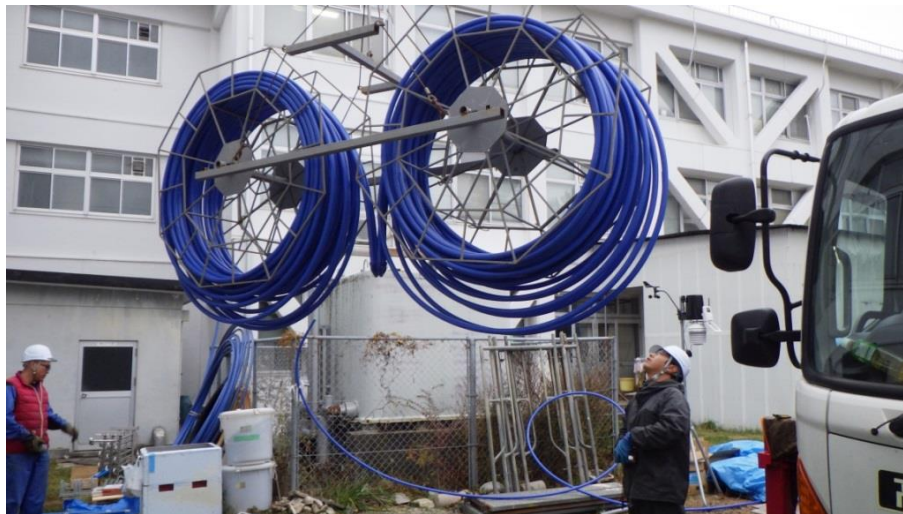
Fig. 3-5 U-tube installation process.
