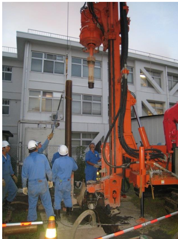
Fig. 3-3 Rotary drilling equipment.
