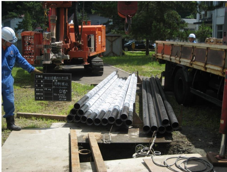
Fig. 3-4 Casings for GHEs.
