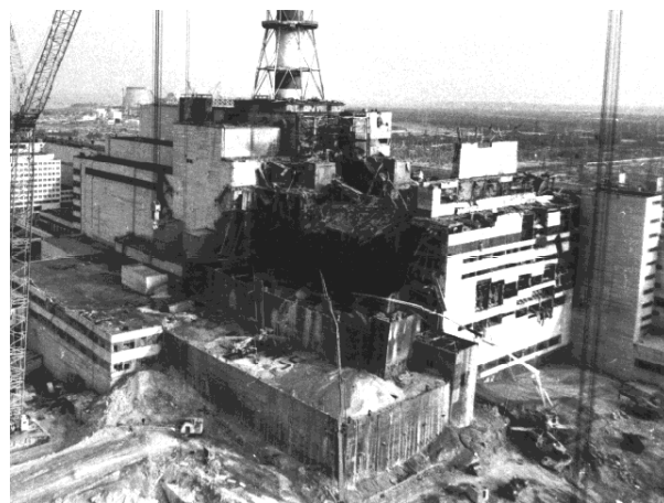
Figure 4-2. Aerial View of the Damaged Chernobyl Reactor Facility (adapted from http://193.125.172.36/www-klae/POLYN/history.html )
