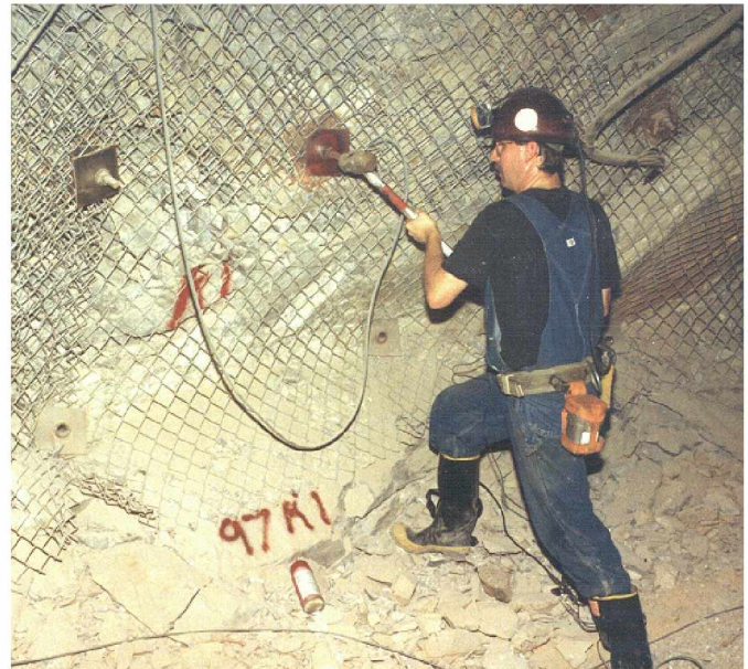
Figure 5.—Creating a source of seismic waves.
