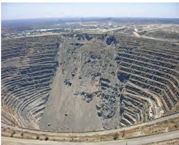
Figure 6.—Slope failure in Palabora pit (left) induced by cave from underground mine (right).
