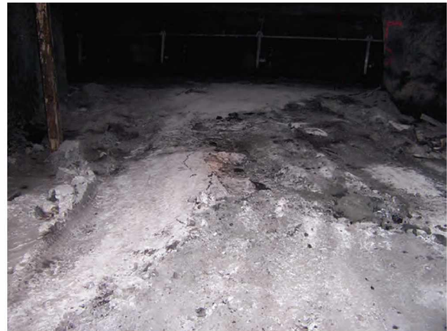
Figure 4.—Localized floor instability in an Illinois basin coal mine.
