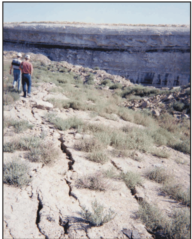
Figure 3.—Cracks near berm of spoil pile can create hazards for trucks dumping material near edge.
