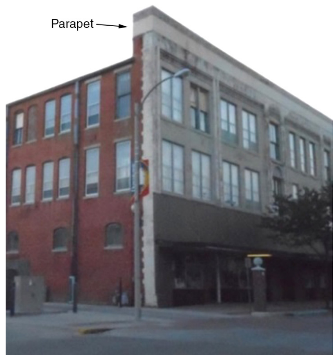
Photo 1. Building with parapet wall (Courtesy of Buildingsonfire.com)
