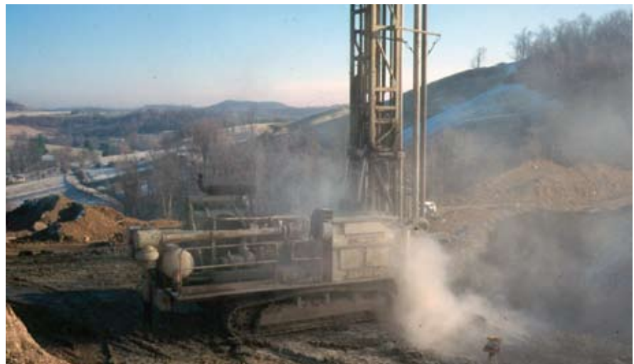
Figure 1. Rock drilling without appropriate dust control.
