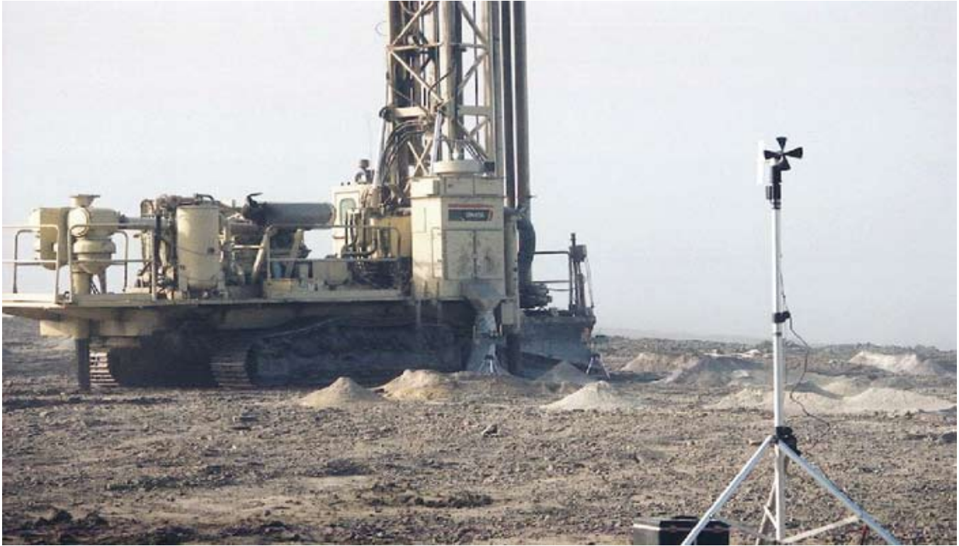
Figure 2. Dry dust control system working correctly.
