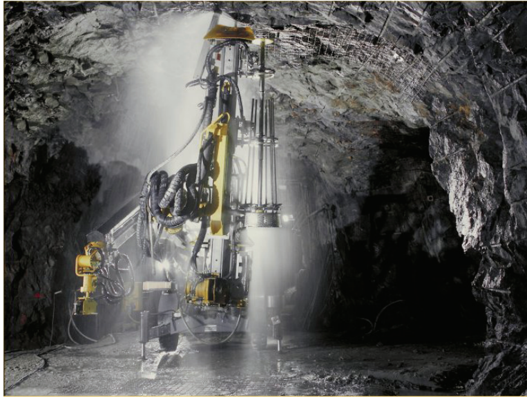
Figure 10 - Drill used to install rock reinforcement.
