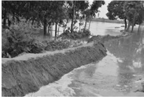
Figure 3. Building Levees to Prevent Floodwater
