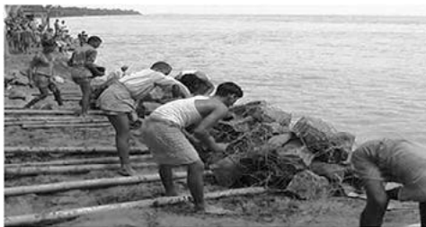
Figure 4. Laying of Boulders to Check Water and Land Erosion
