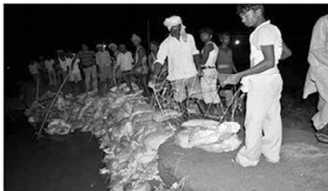
Figure 2. Laying Sandbags to Check Spread of Floodwater
