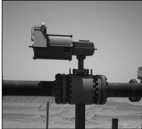
Figure 23: Check Valve, Nasiriyah Degassing Station
