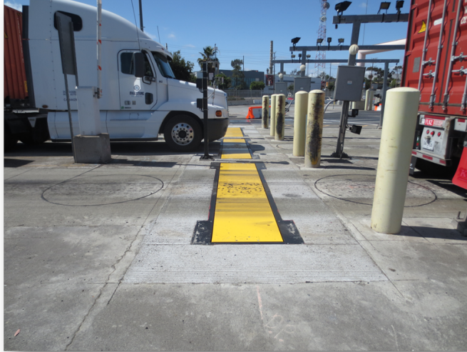
Figure 1.11: Road Vehicle Weigh-In-Motion [15]. © 2016 Intercomp.
