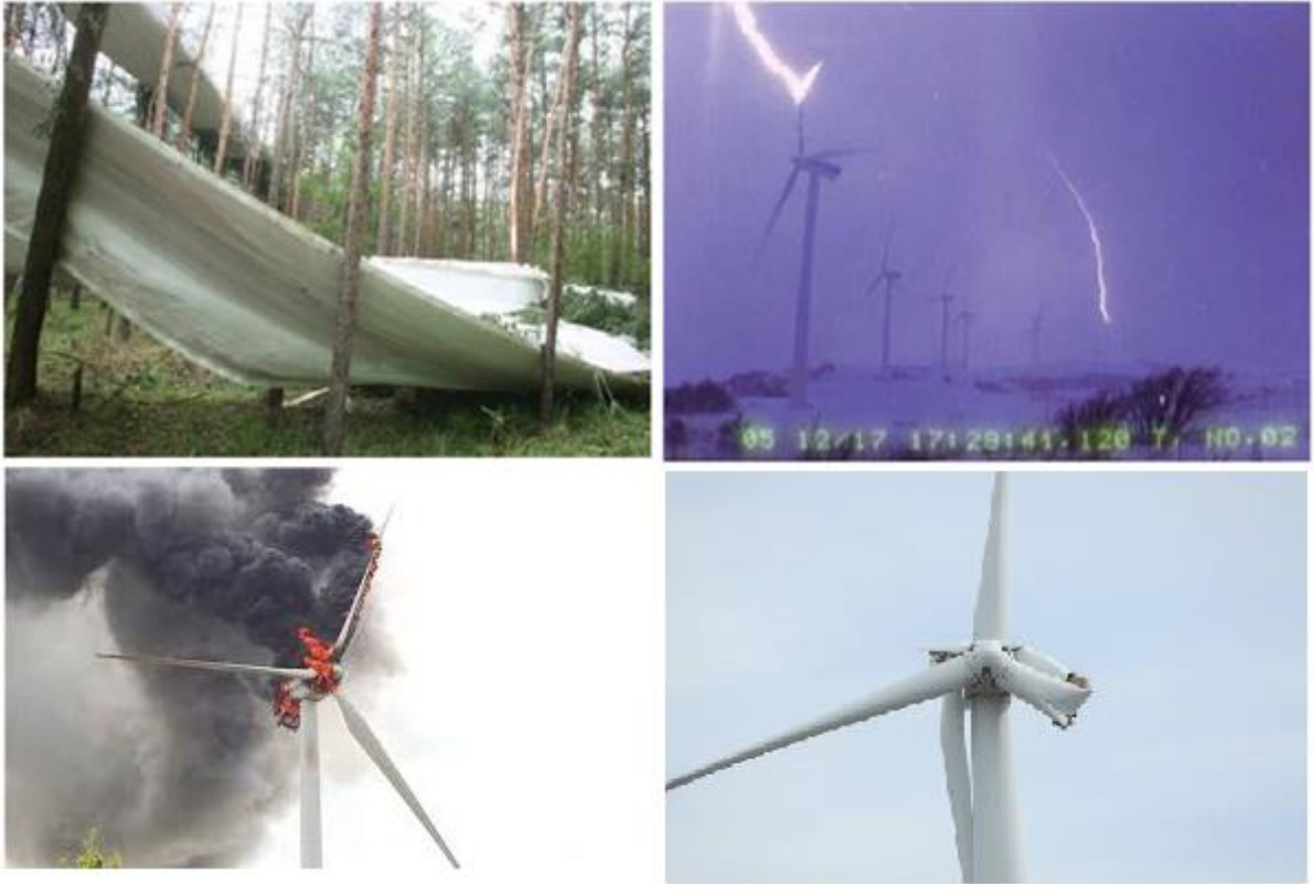
Fig. 1.2: Wind, high load, or lightning strike induced broken, damaged, or burned blades (Adapted from Ref. [16])
