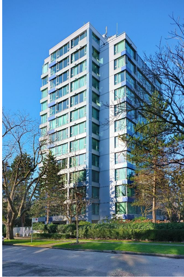
Figure 3-1: The Belmont as viewed from the north-east corner in February 2013. Provided by RDH.
