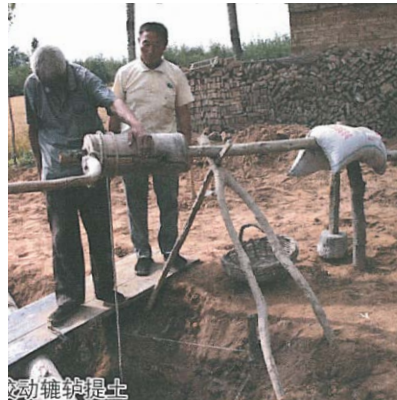
FIG 3.39 Excavation of deep earth with a lu-lu
