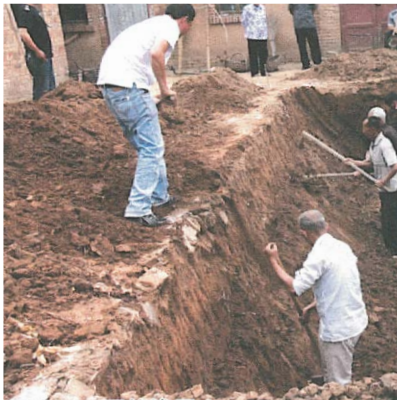
FIG 3.38 Excavation of shallow earth
