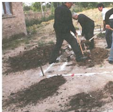
FIG 3.33 Pray before construction FIG 3.34 Construction starts
