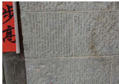
FIG 3.65 Detail of Stone facade in Shanxi
