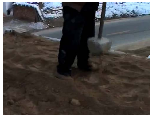
FIG 3.71 Packing down the Yao-dong foundations
