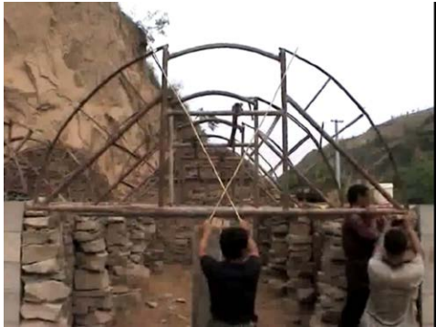
FIG 3.25 Framing the arched roof, calculating the arrows- building the vault
