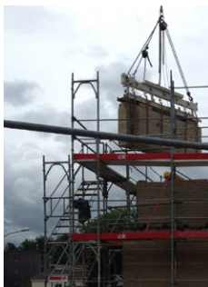
FIG 8.1 Basehabitat workshop lecture by Martin Rauch, and field trip picture
