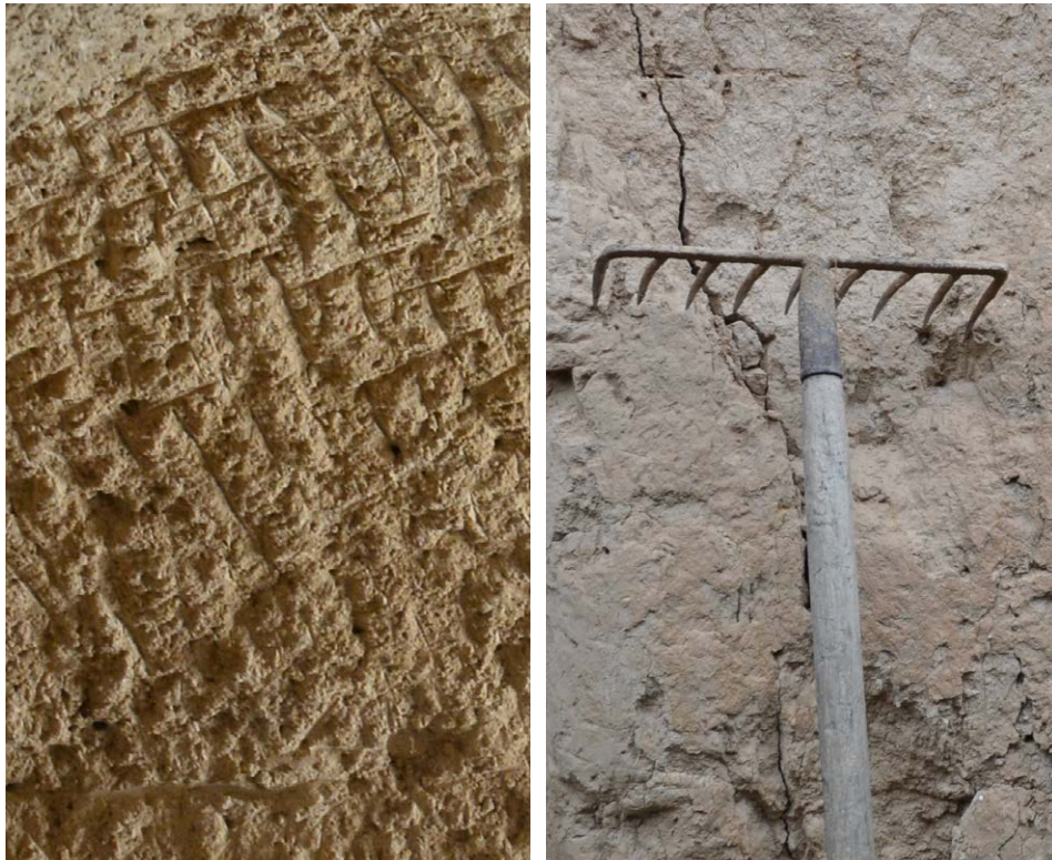
FIG 3.42 texture of loess wall and a “Si-zua-pa” (four claw iron rake)
