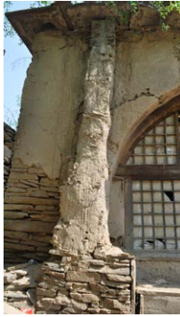
FIG 7.76 yao-dong chimney in Guo-family village, Mizhi
