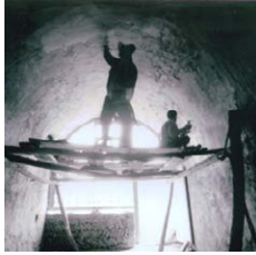
FIG 3.68 Shanbei Above-ground Yao-dong
