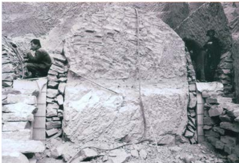
FIG 3.70 Shanbei Above-ground Yao-dong
