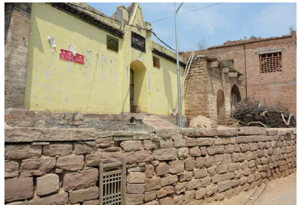
FIG 5.26 School in Gou-di village, Shanxi
