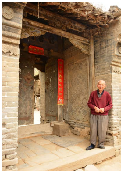
FIG 3.75 Yao-dong entrance in Xi-guo-village, Henan Yao-dong entrance in Gou-di village, Shanxi Yao-dong entrance in Mu-tou-yu Village, Shanbei
