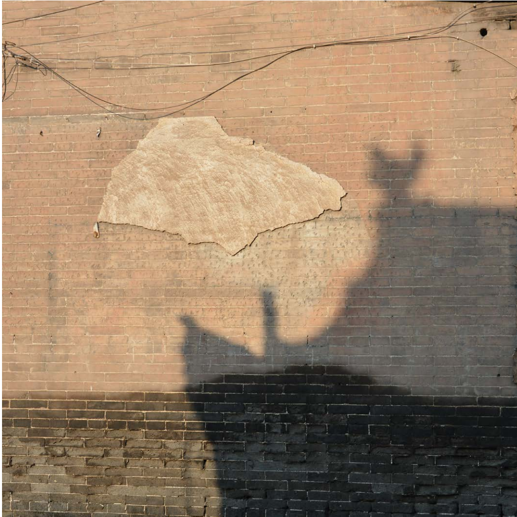
FIG 4.9 Wall in Ping-yao
