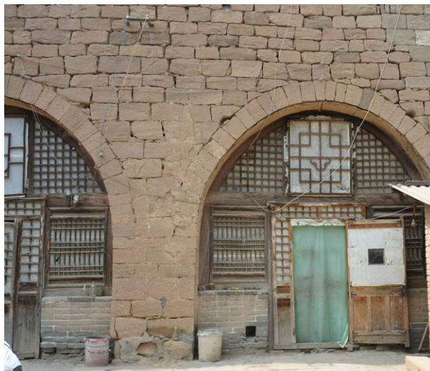
FIG 3.58 yao-dong made of bricks in Ping-yao yao-dong made of stones in Mu-tou-yu village
