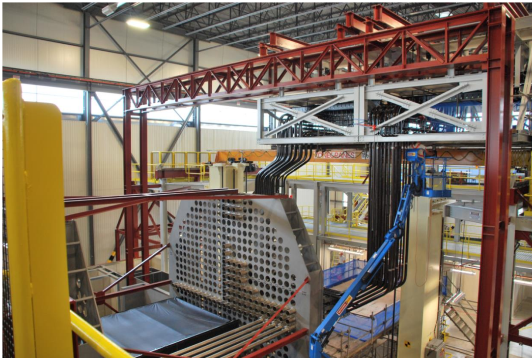
Figure 2-1: Nuclear reactor training mock-up with reactor face, fuel channels, and upper and lower feeders visible
