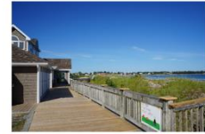
Vulnerable infrastructure, Lockeport, NS
