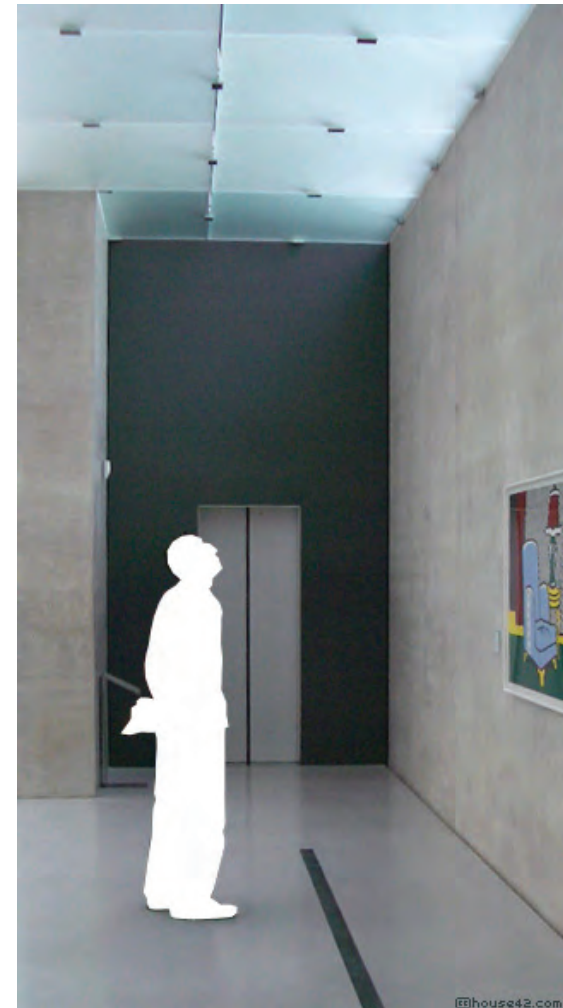
Figure 3-48 Scale of the building is obscured by the ceiling finish that allows daylight to penetrate the four sides of the building.
