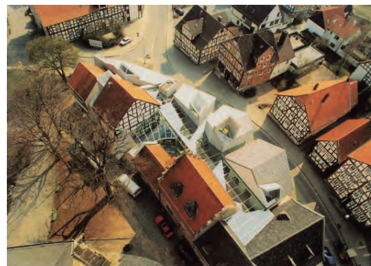
Figure 3-21 View of the Korbach Museum from the tower of St. Kilian.
