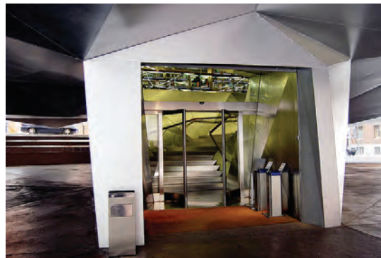
Figure 3-52 Entrance from grade level from below the building structure of the CaixaForum Madrid.
