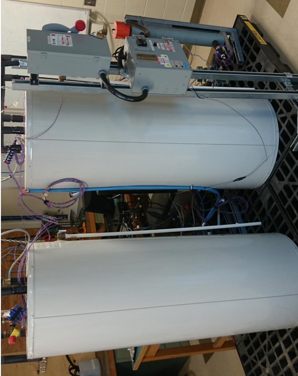
Figure A.2 – DHW tank (left) and float tank (right) with thermocouple instrumentation (centre)
