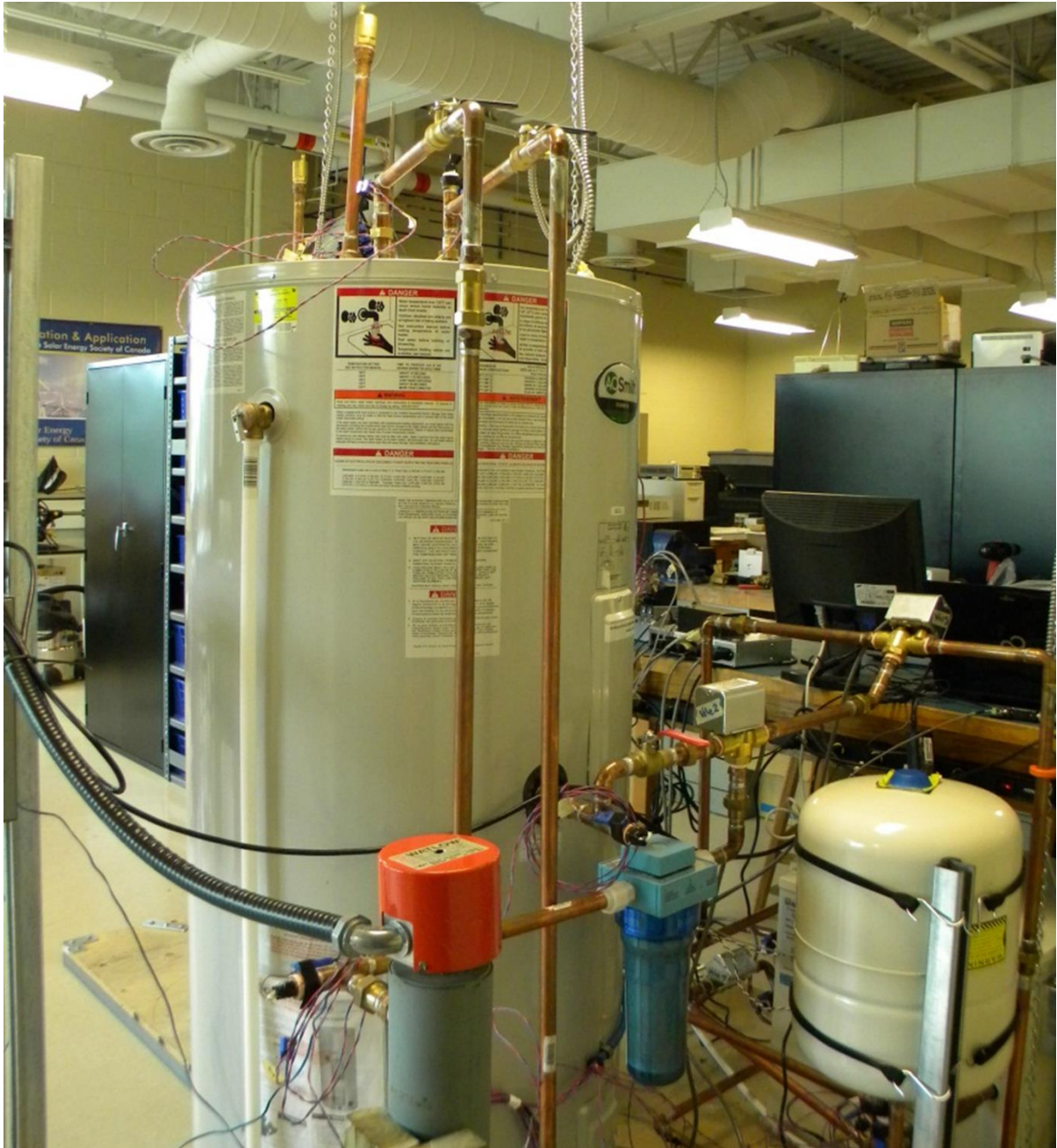
Figure A.1 – Partial view of experimental apparatus before pipe insulation
