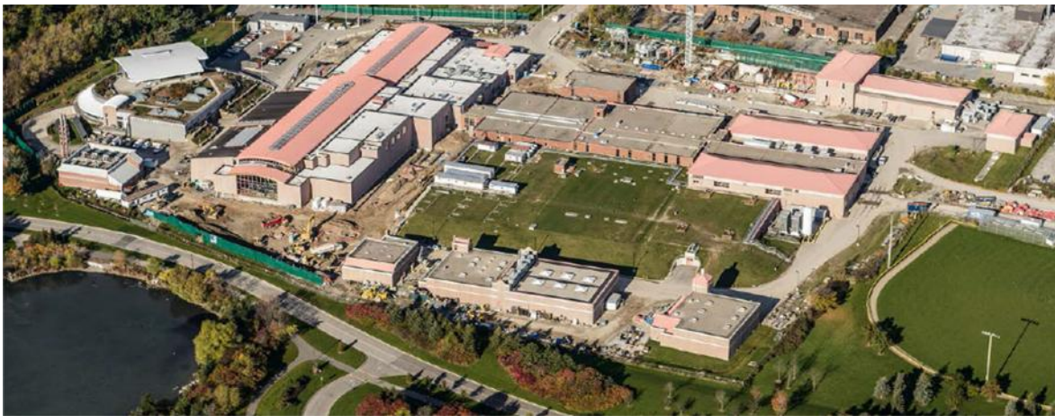
Figure 3.1 The Lakeview WTP aerial photo. (Reprinted with permission from the Region of Peel, 2013)
