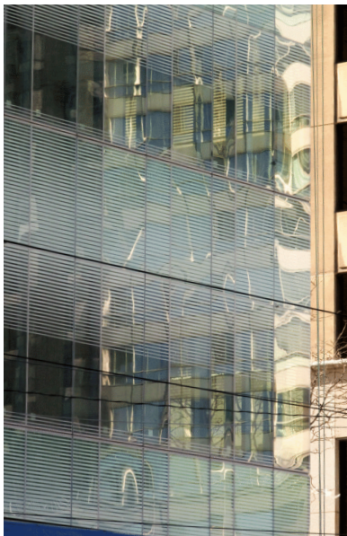
2-14 SickKids Hospital: Peter Gilgan Centre for Research and Learning (Diamond and Schmitt Architects, urbantoronto.ca , 2013)
