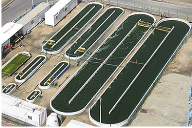
1-30 Open pond bioreactor. (Seabiotic, 2006)
