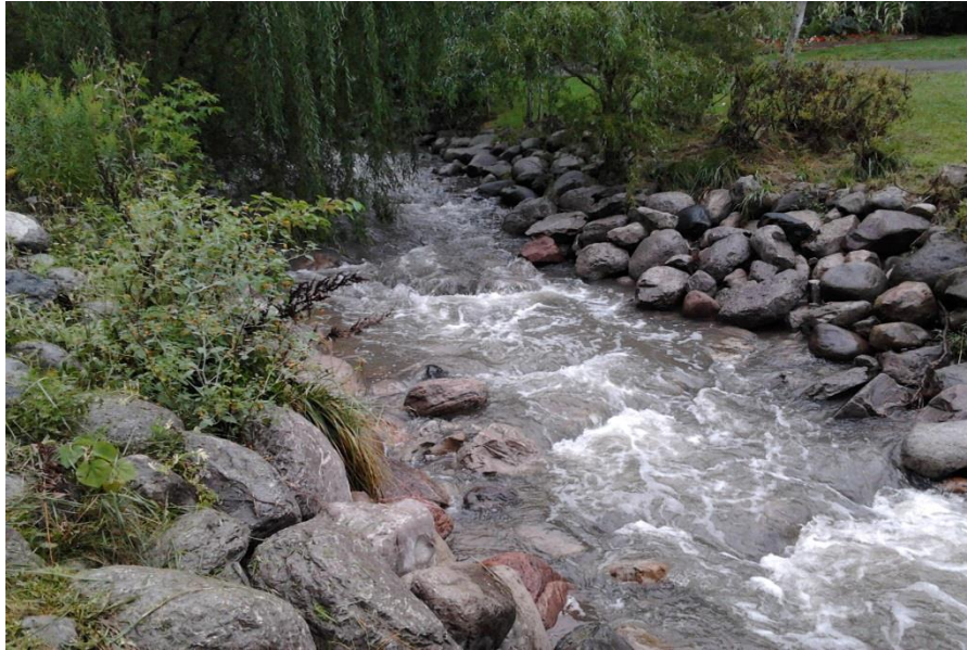
Figure 31. Wilket Creek near pebble count Site S3 A showing engineered banks with large particles sizes.
