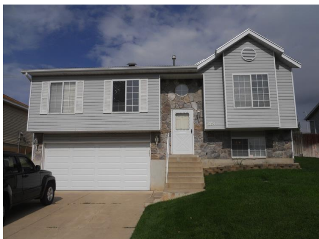
Figure 2-2: Front view of ASU vapor research house in Layton, UT
