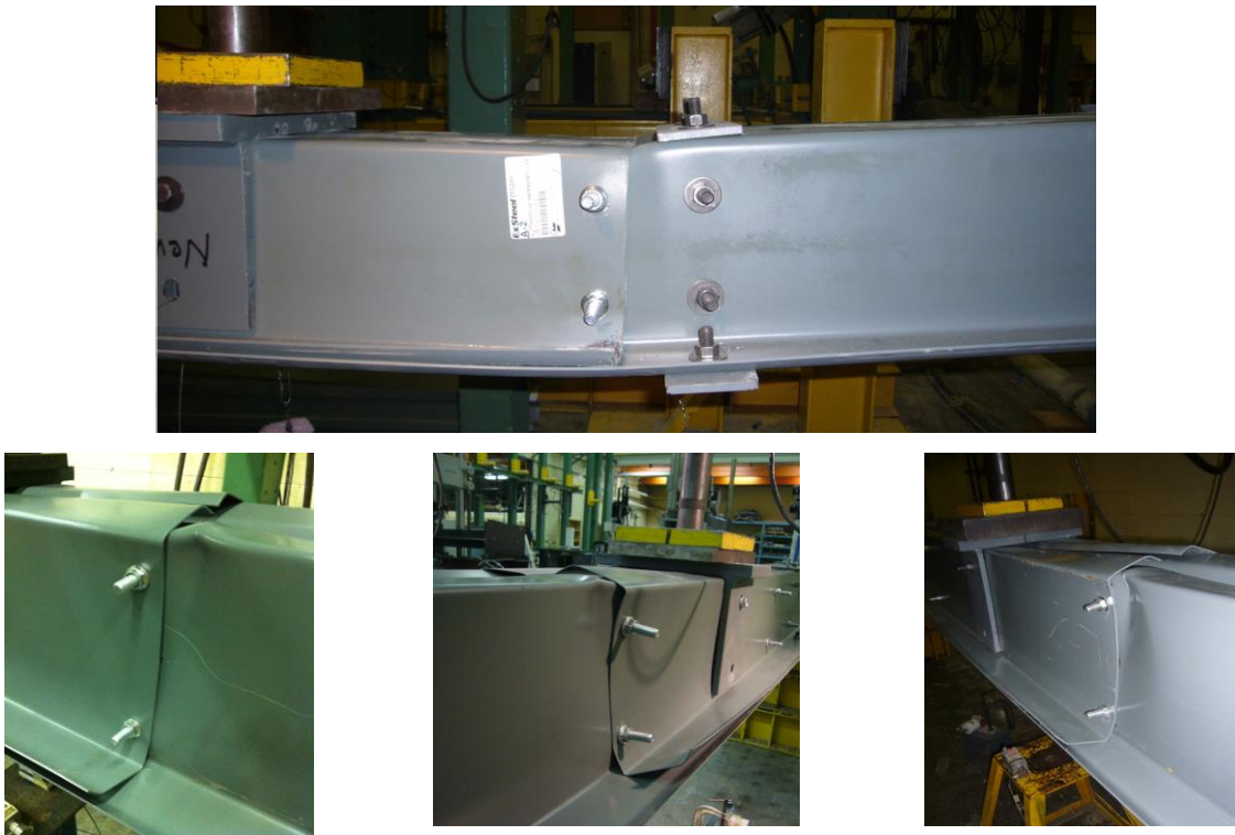
Figure 4-2 Photograph of Typical Failure Mode at the End of Lapped Connection
