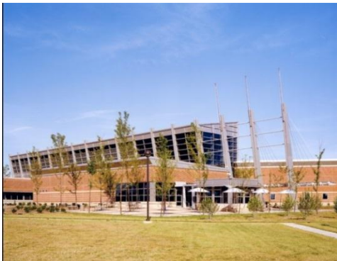
Figure 3.3: A TRACON facility. Adapted from (K. Dixon Architecture PLLC, 2012)
