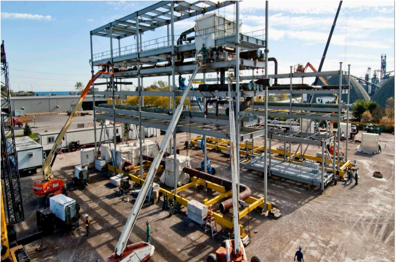
Figure 5-10: Example of the Value Unit: Piping Module
