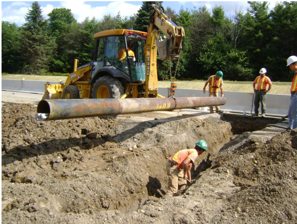
Figure 3-10: Conduit Installation
