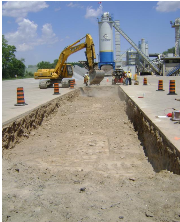
Figure 3-15: Opening the Trench to Construct the Perpetual Pavement Section
