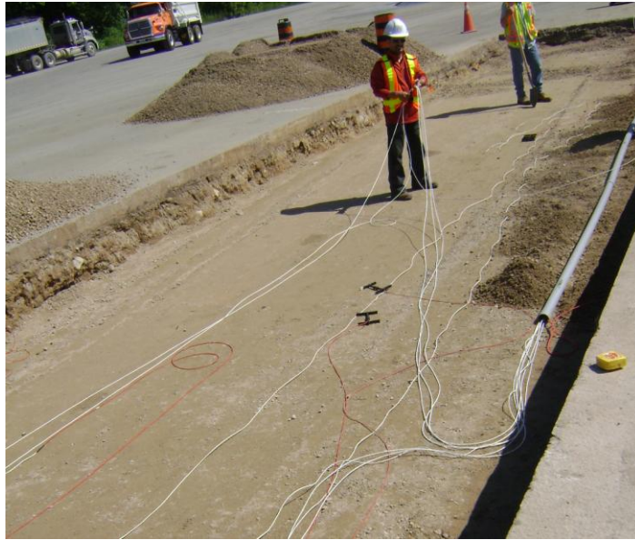
Figure 3-16: Preparation for ASG Installation on Top of Granular A
