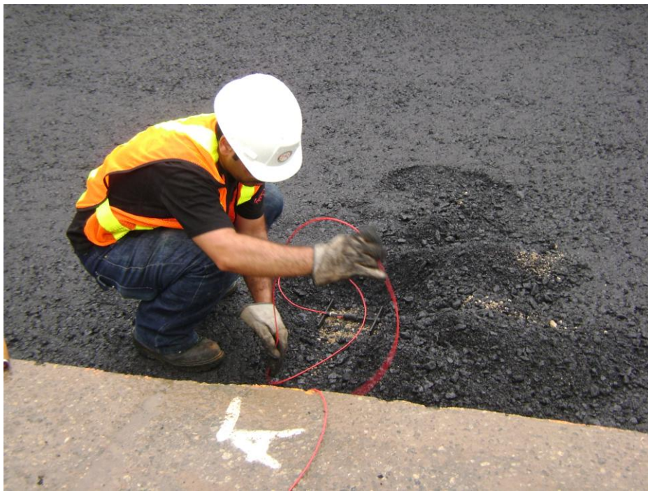
Figure 3-17: Installation of ASG at the Bottom of RBM Layer
