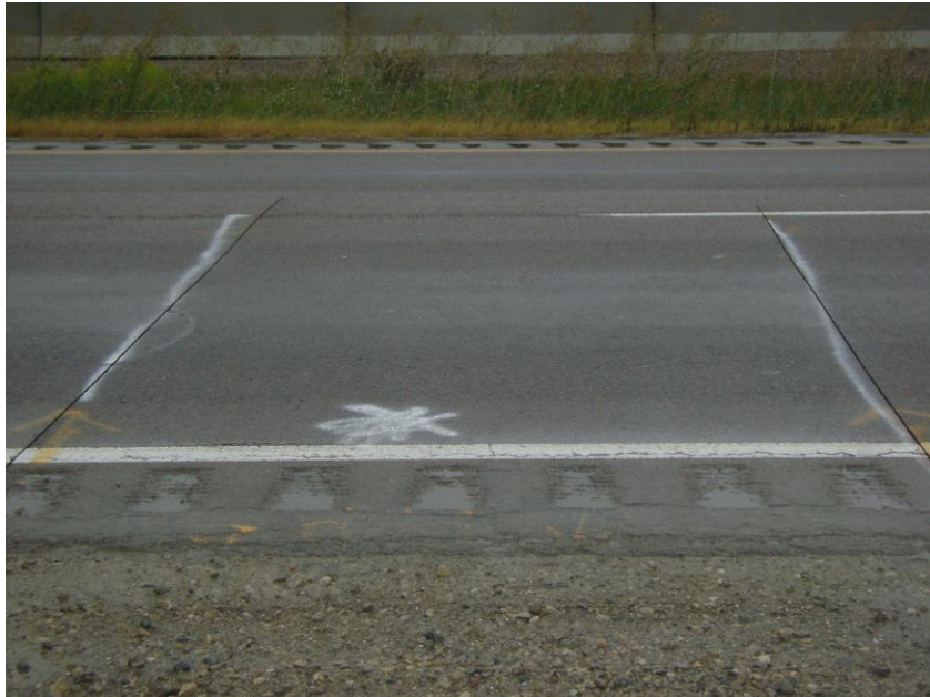
Figure 3-9: Paving Marking Prior to Open Trench Excavation
