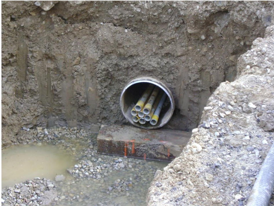
Figure 3-11: PVC Tubes Inside the Steel Conduit
