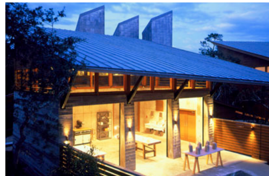
Figure 2.16 The sculpture studio at ACA boasts an outdoor work area linked to the interior space by three roll-up doors, and sheltered by the large roof overhang creating quite a strong blurring of indoor and outdoor space for the artists to use.
