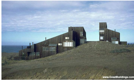
Figure 5.1 SR Elevation Photo
