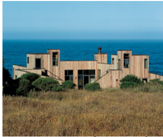
Figure 5.2 SR Elevation Photo
