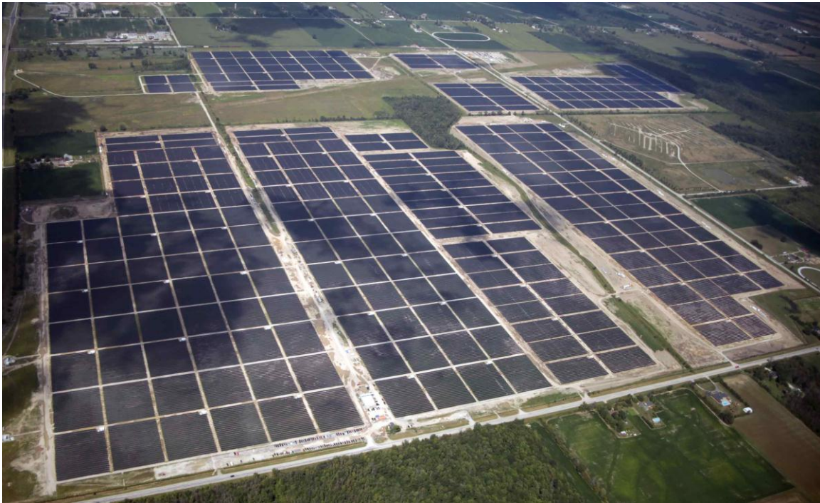
Figure 1-4: Clouds partial shading in Sarnia PV farm
