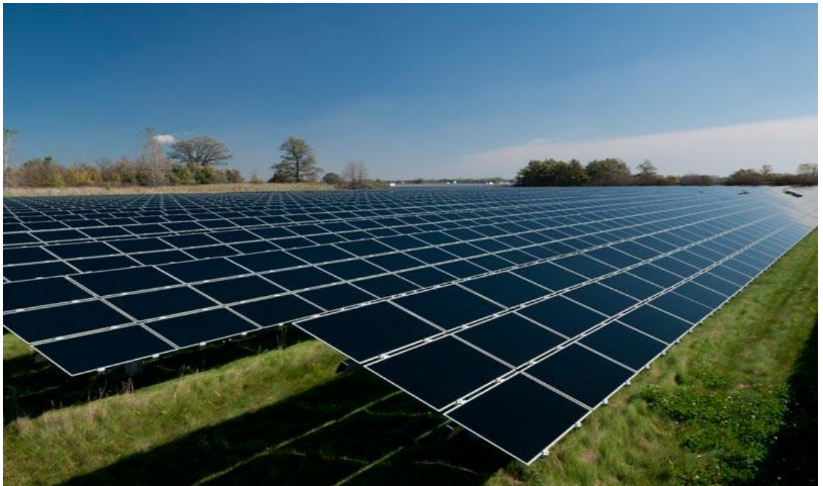
Figure 1-6: Sarnia PV farm is installed on a large area and in landscape to avoid array partial shading
