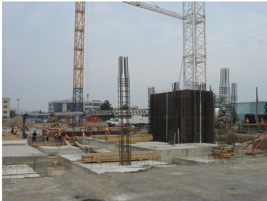
Figure 6.8 Column rebar at Engineering V Building Site
