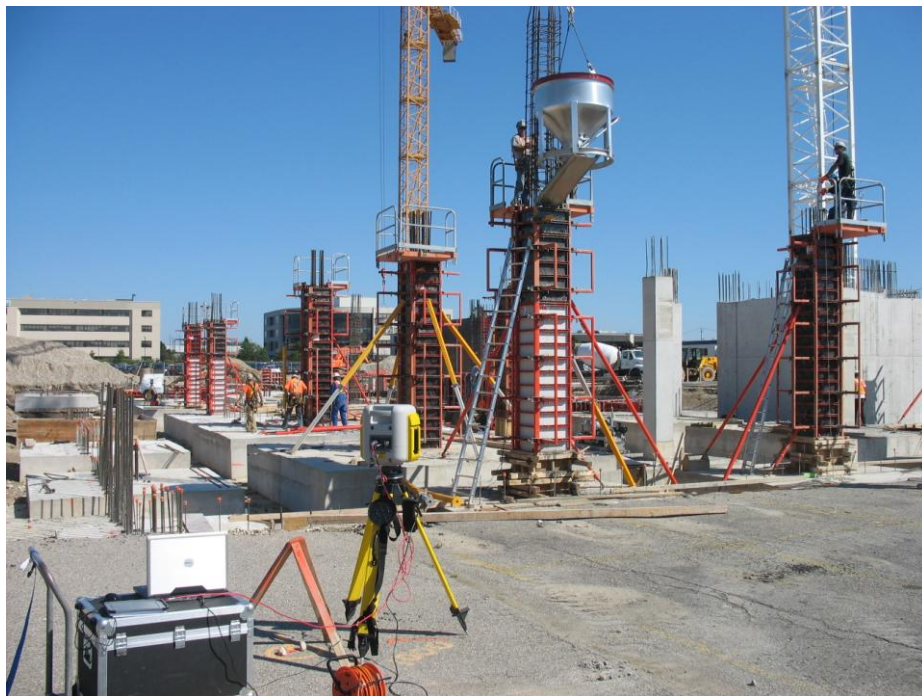
Figure 6.1 Temporary objects at E5 Building site – July 25, 2008
