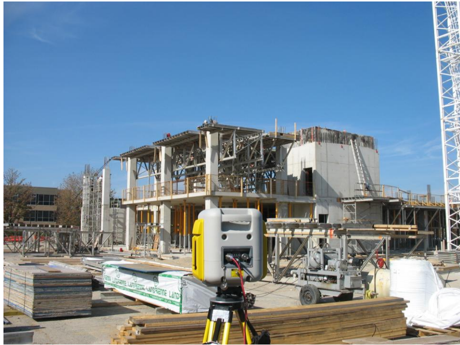
Figure 3.3 Scanning at E5 Building construction site on September 26, 2008
