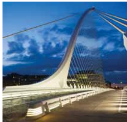
image 3.20 samuel beckett bridge, dublin santiago calatrava
