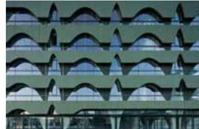
pre-fabricated painted concrete façade elements
